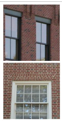
Figure 23-423.f.3.iii.a Headers Steel Lintel (above) and Brick Jack Arch (below)
