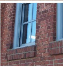
Figure 23-423.f.3.iii.b Sills Cast Concrete (above) and Brick (below)
