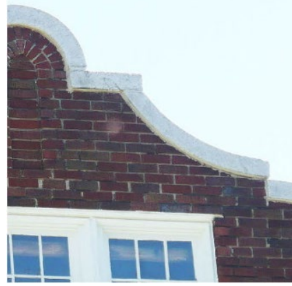
Figure 23-423.f.3.iii.c Caps Concrete Pier (above) and Cast Stone Cornice (below)
