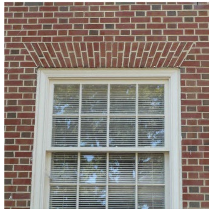
Figure 23-423.f.3.iii.a Headers Steel Lintel (above) and Brick Jack Arch (below)
